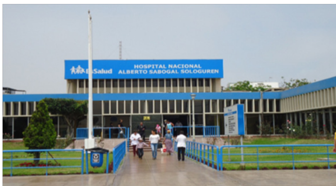
Figure 3 ESSALUD: Peruvian hospital network where nanomafias would operate. 6
